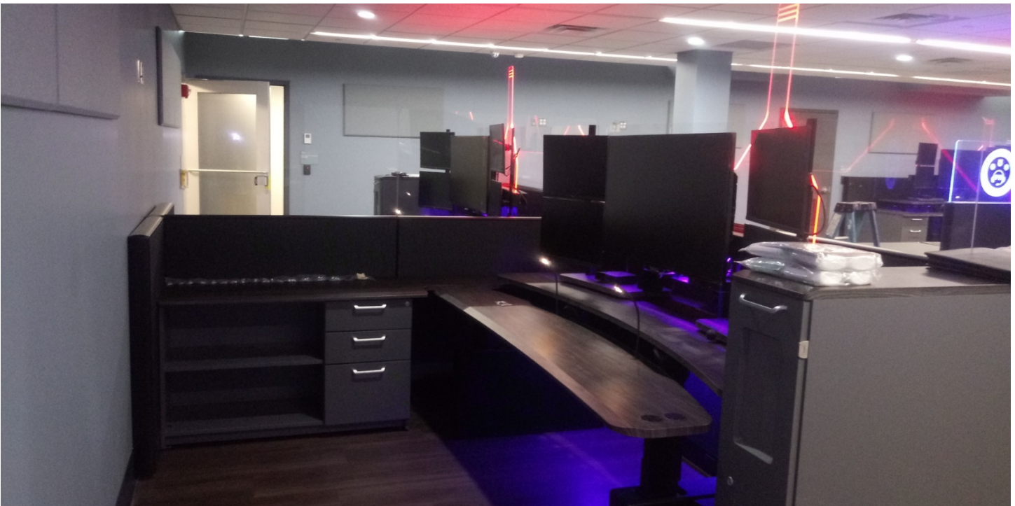
Dispatch 120 – Xybix workstation & computer equipment installations continue.
