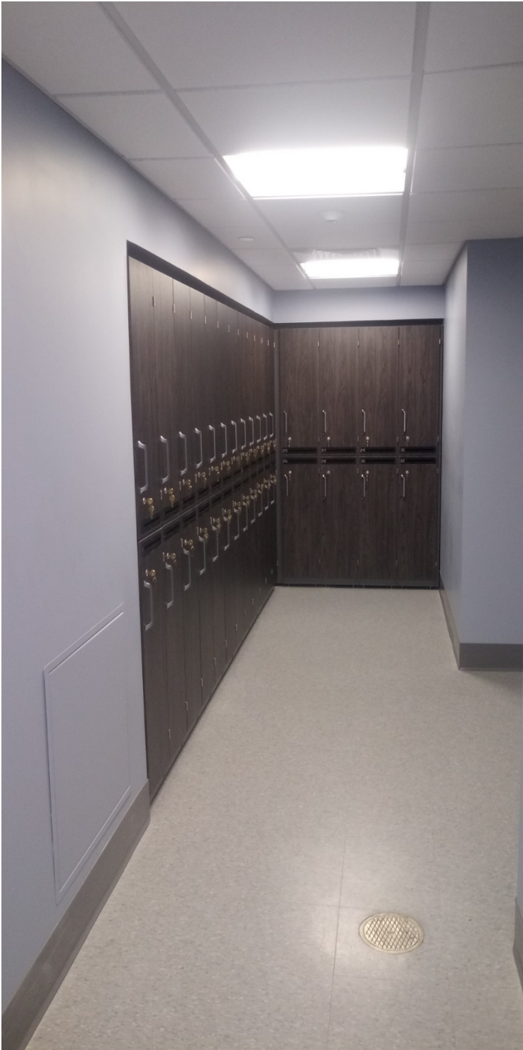
Corr. 018 – Lockers installed.
