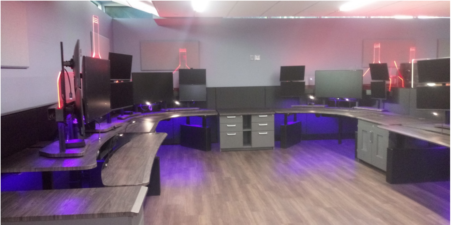
Dispatch 120 – Xybix workstation & computer equipment installations continue.
