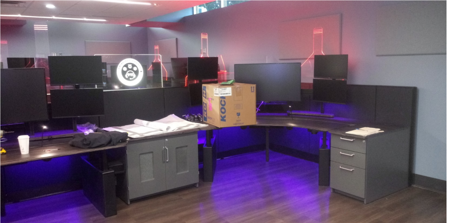
Dispatch 120 – Xybix workstation & computer equipment installations continue.
